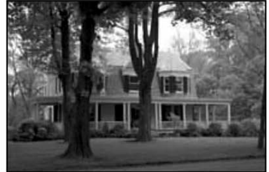
This 1897 house is one of several in Sudbrook Park designed by Baltimore architect George Archer.
